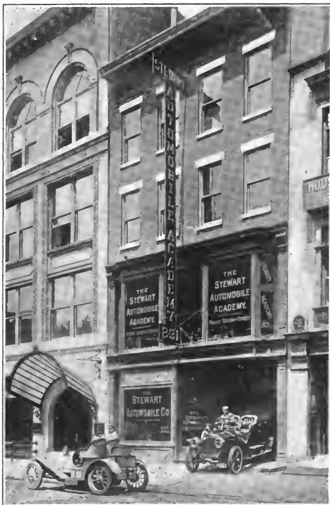
Exterior of Stewart Garage, New York City
